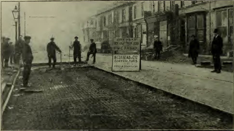
CONCRETE ROAD AT MIDDLESBROUGH.
